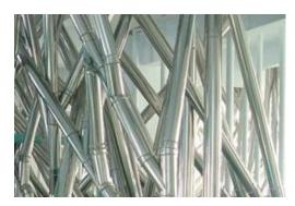
Gravity Spouting is used in a wide range of flour/feed and related material handling installations
